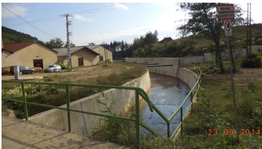
Figure 5. Completed retaining wall (Recsk, Mining Site I-Lahóca, 23/09/2014)
