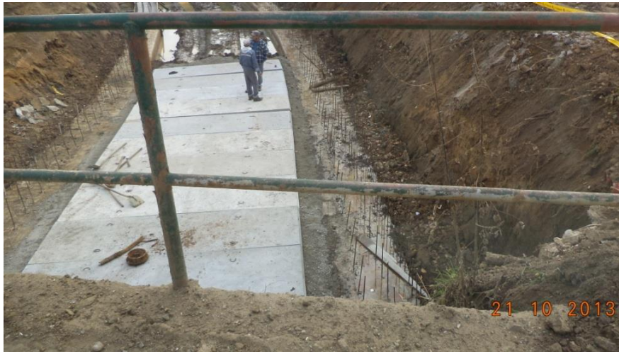
Figure 4. The works of retaining wall (Recsk, Mining Site I-Lahóca, 21/10/2013)
