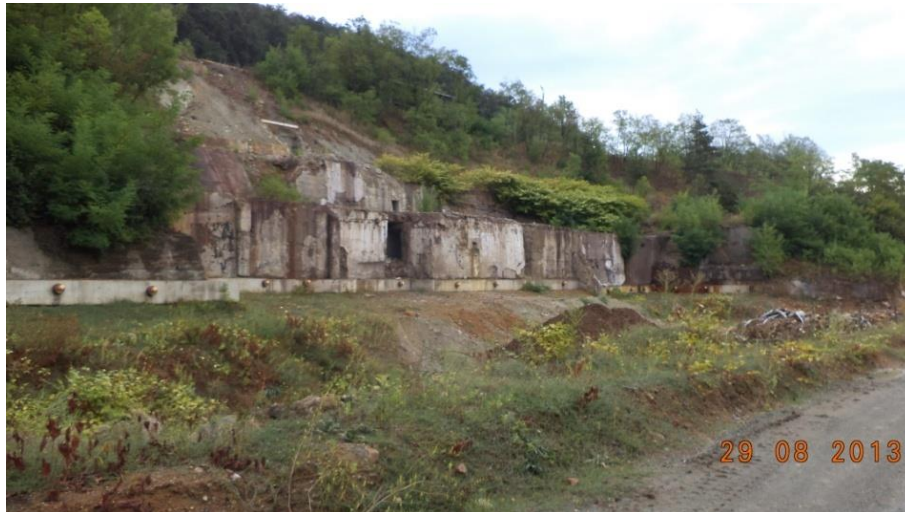
Figure 6. Ruins of the ore dressing building (Recsk, Mining Site I-Lahóca, 29/08/2013) Source: Own photo
